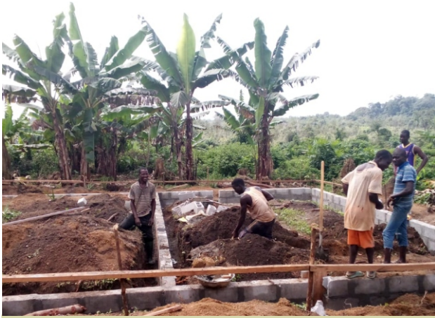
Construction has Begun for Panama Women's Group in the Kpanyan District, Sinoe County.
