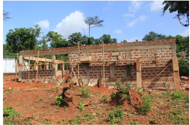
Construction of the Mini Processing Center for Badio's group in Zwedru, Grand Gedeh Nears Roofing
