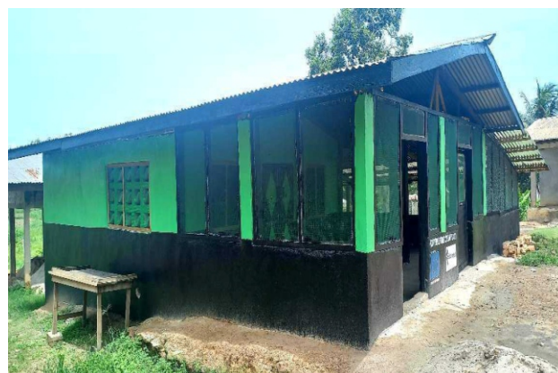
Renovated structure of Faith Temple processing enterprise
