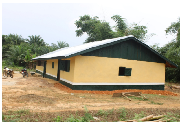
Renovated structure of Agro Green processing enterprise
