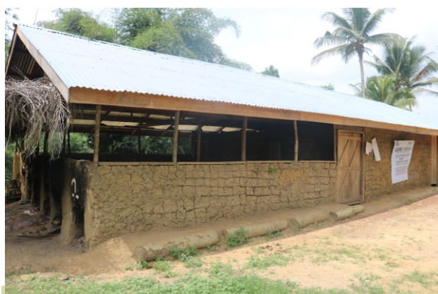
Previous state of Agro Green processing enterprise
