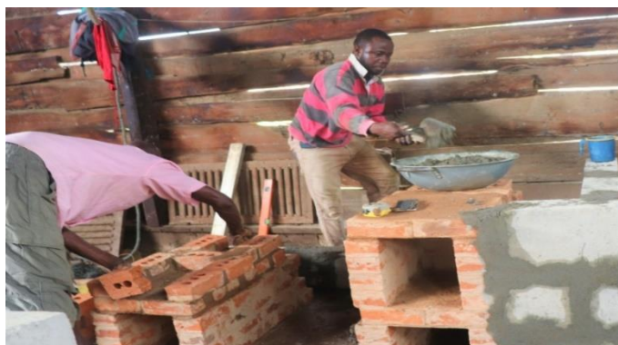
Ahotor oven under construction for a 'stove host' beneficiaries in the Shama Apo community
